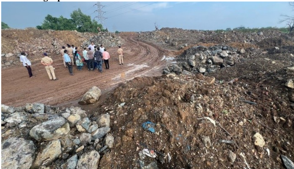
Dumping of debris. C&D waste, Soil, mixed waste partly stabilized.
